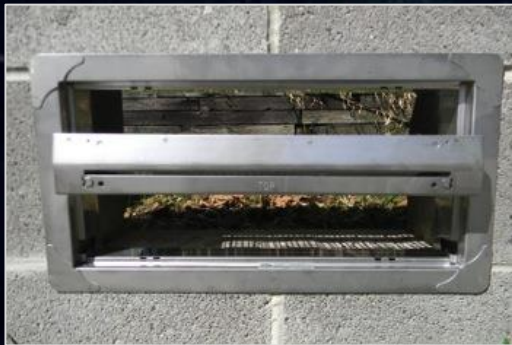
Flood door activated, reveals an un-obstructed opening.
