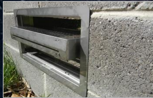
Flood door activated, reveals an un-obstructed opening.
